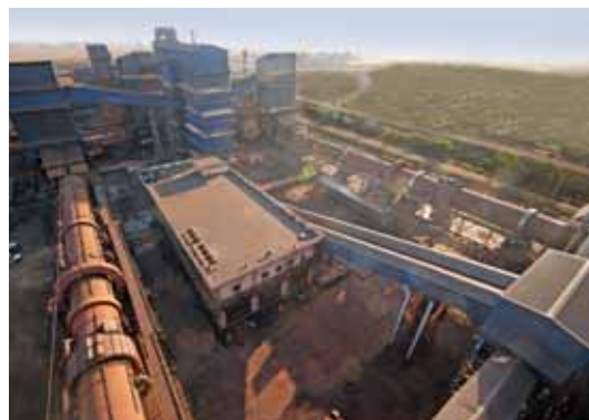
Sponge Iron Plant
